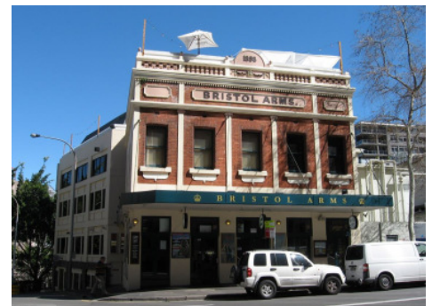
Figure 4.1 East elevation of 81 Sussex Street, the Bristol Arms Hotel
