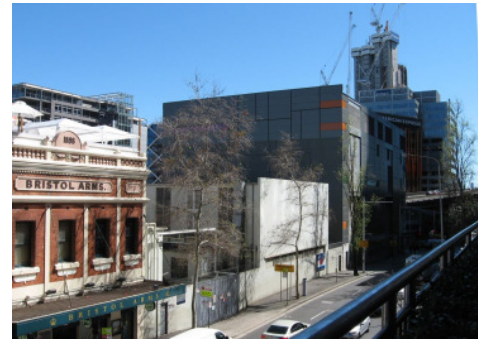
Figure 2.1 The subject site is between the Bristol Arms Hotel on the left and the City North Substation on the right. Note the utilitarian structures on the subject site
