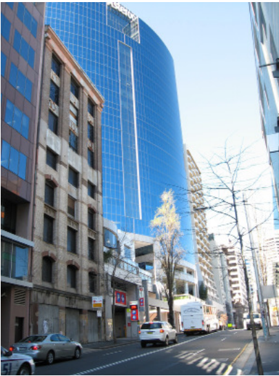
Figure 2.7 Eastern side of Sussex Street with the glazed commercial tower opposite the subject site
