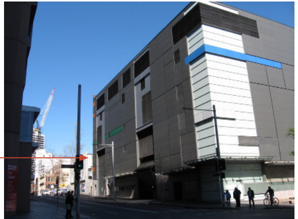
Figure 2.8 Western side of Sussex Street on the corner with Erskine Street, with the Substation on the right, next to the subject site
