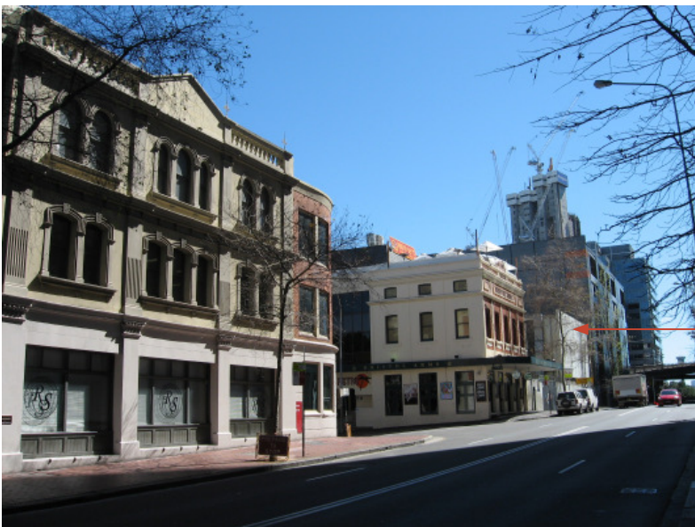
Subject site at 65-79 Sussex Street
