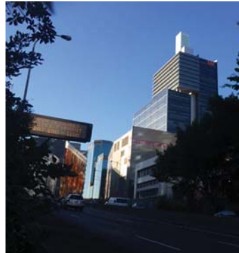
WESTERN DISTRIBUTOR VIEW NORTH
