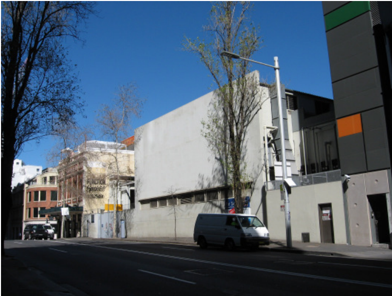
Figure 2.3 The existing structures on the subject site at 65-79 Sussex Street, with the Bristol Arms Hotel on the left and the Substation on the right
